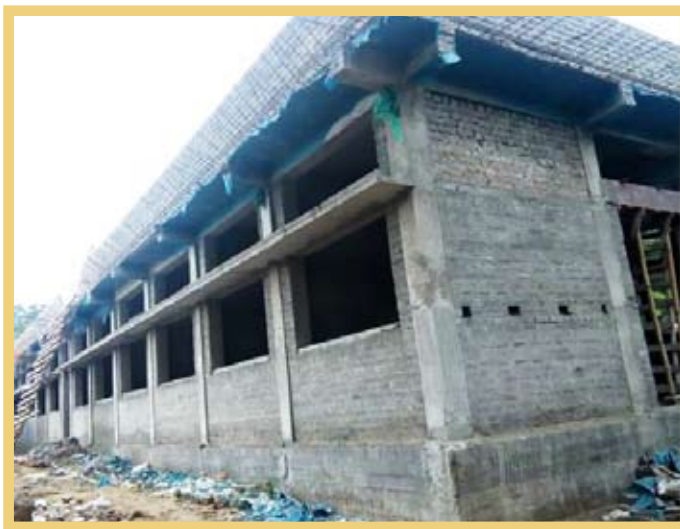
Construction of Fish Market, at Danipalli, Sambalpur
