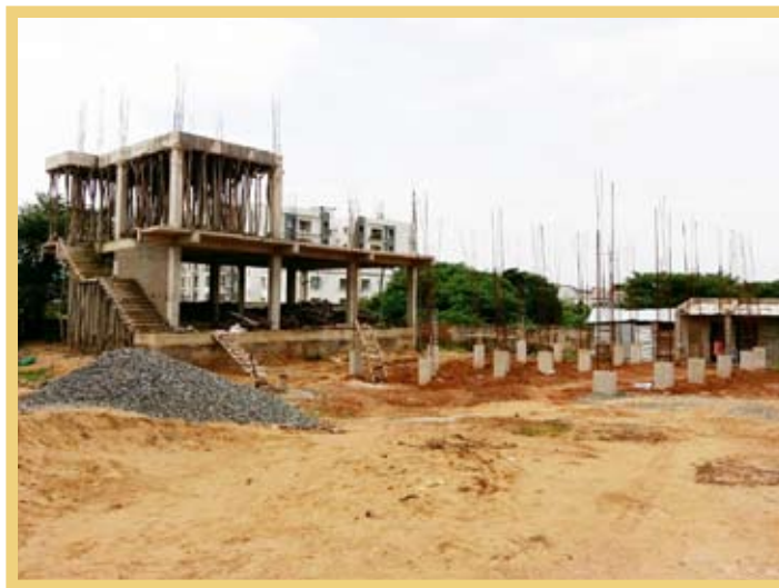
Construction of Modern Abattoir at Gadakana, Bhubaneswar
