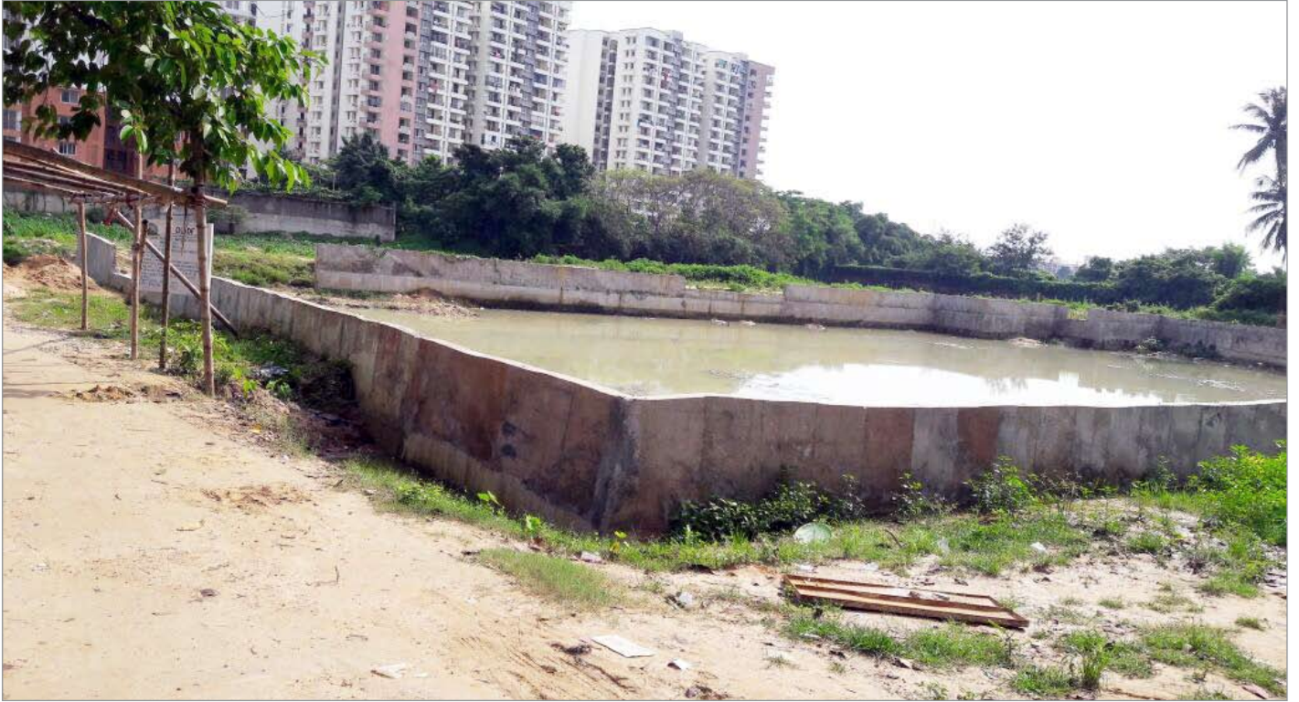
Reclamation of Jhara Pokhari, Bhubaneswar (Construction Ongoing)
