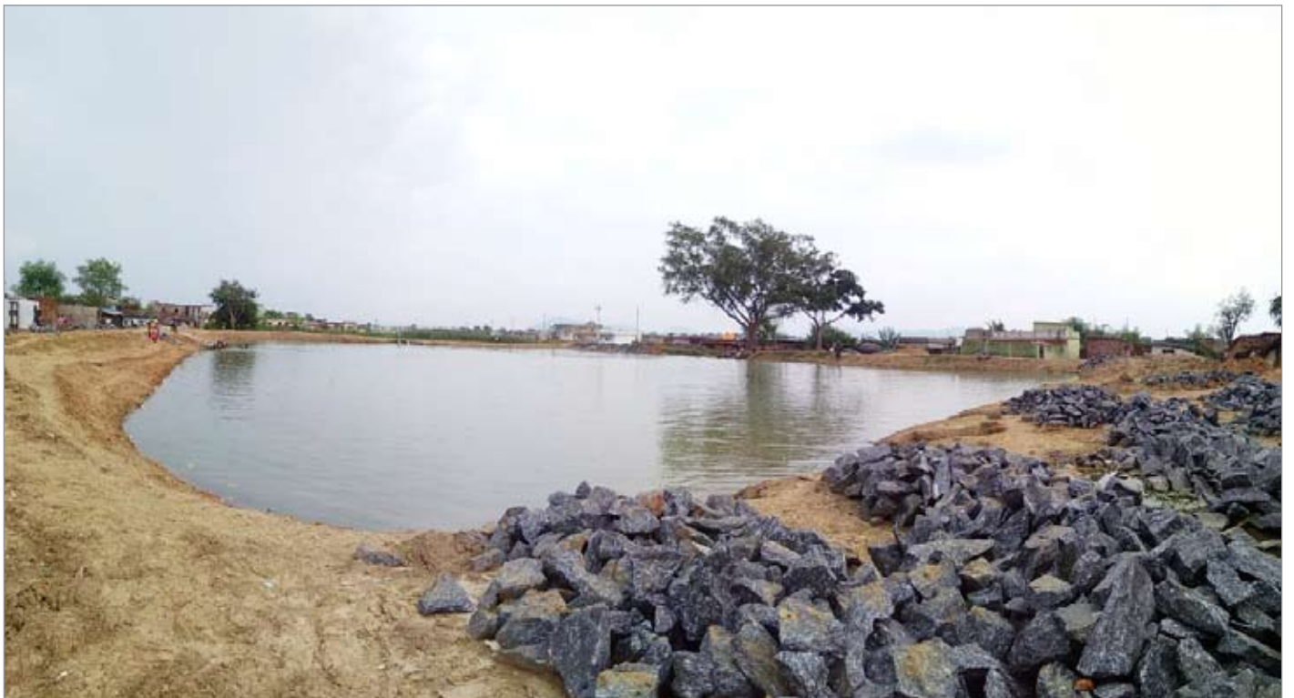
Reclamation of Motijharan Pond at Sambalpur (Construction Ongoing)
