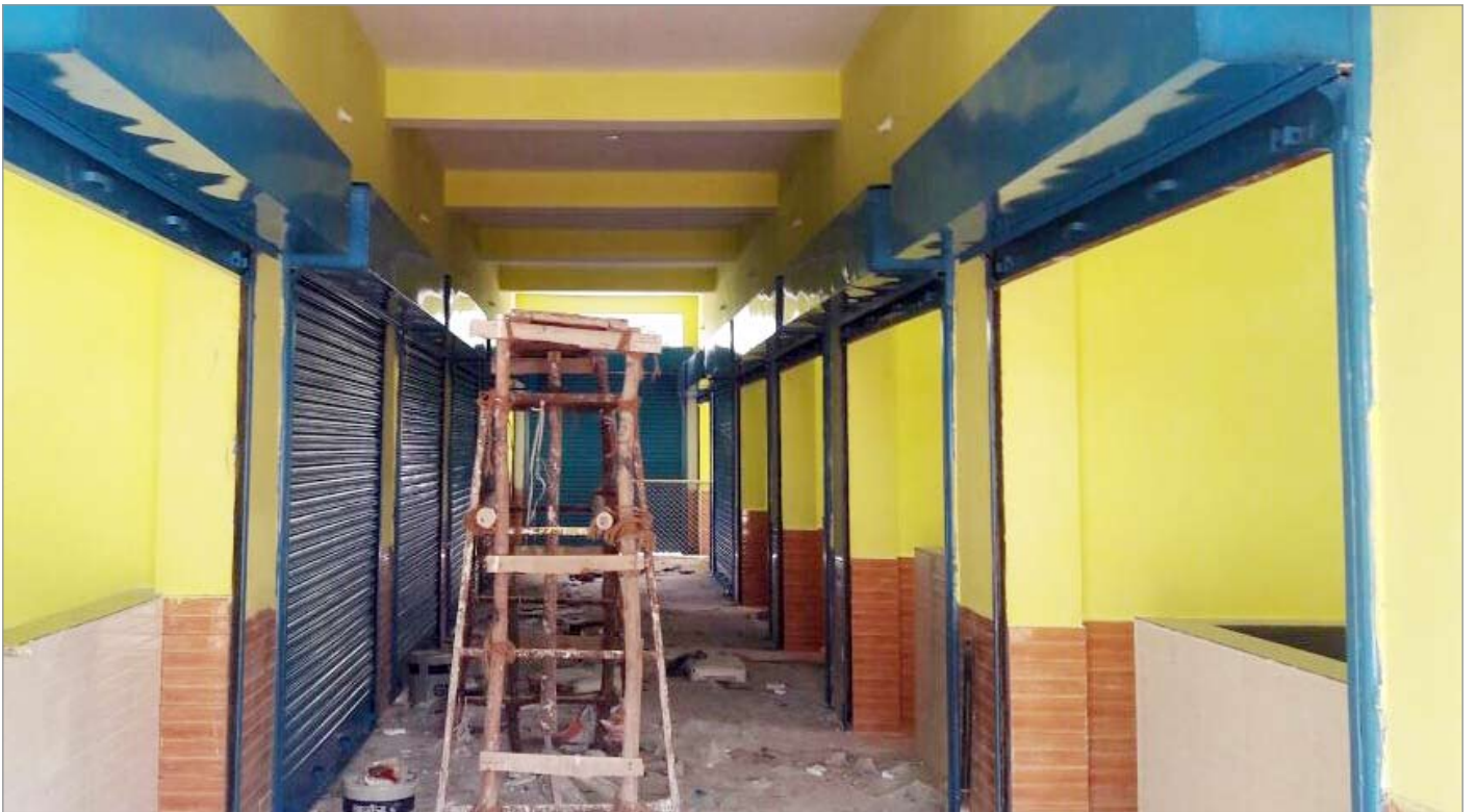
Fish Market at Kamlibazar in Sambalpur (Nearing Completion)
