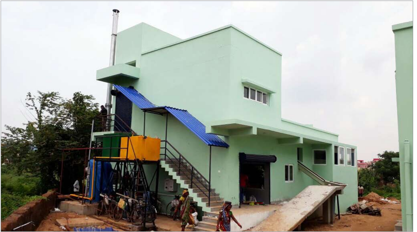
Administrative Building of Modern Abattoir, Gadakana, Bhubaneswar (Nearing Completion)
