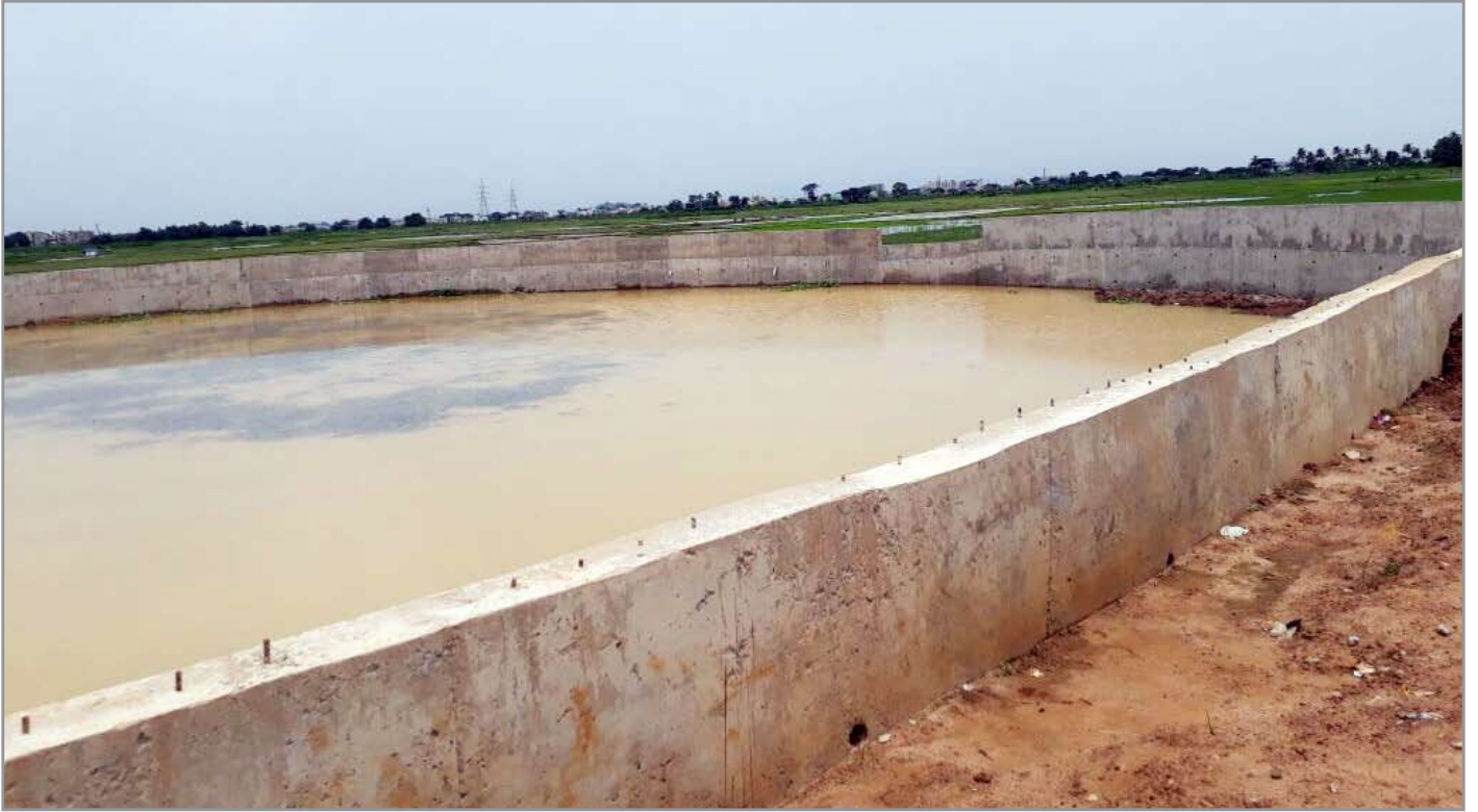
Reclamation of Bagua Tank, Bhubaneswar (Construction Ongoing)
