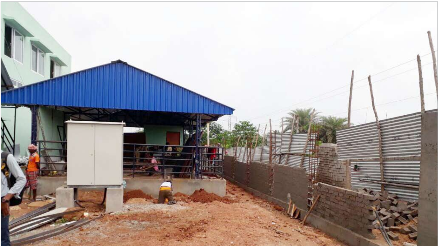
Lairage of Modern Abattoir, Gadakana, Bhubaneswar (Nearing Completion)
