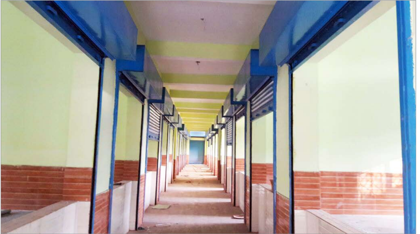
Fish Market at Danipalli in Sambalpur (Nearing Completion)
