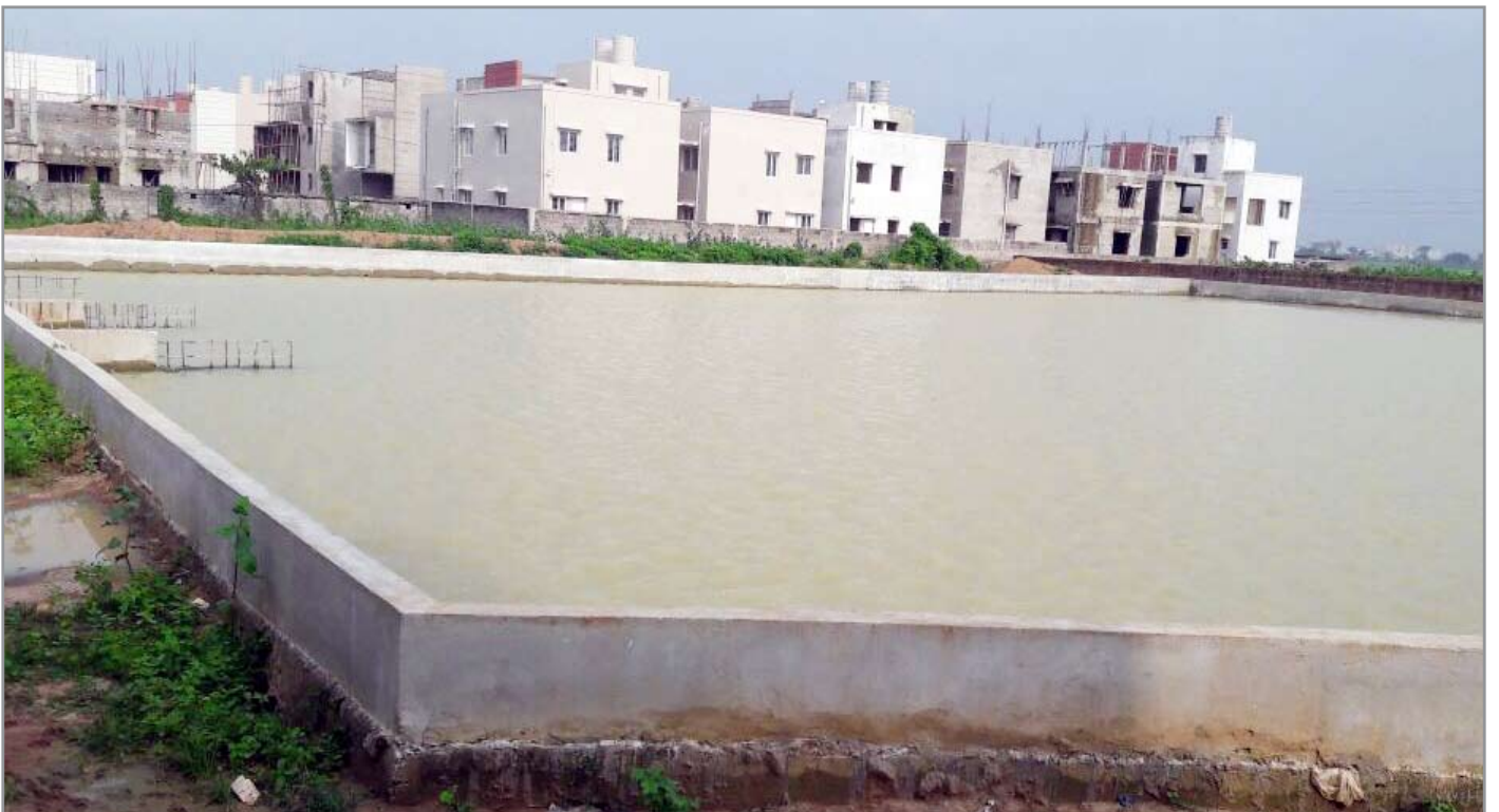
Reclamation of Badapokhari Pond, Bhubaneswar (Construction Ongoing)
