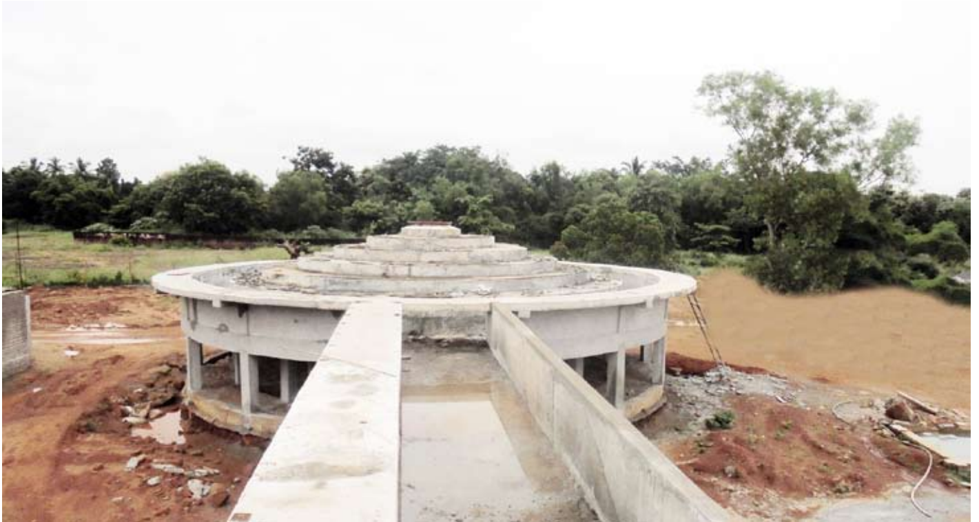
Aerator cum Bypass Channel (Construction Ongoing)
