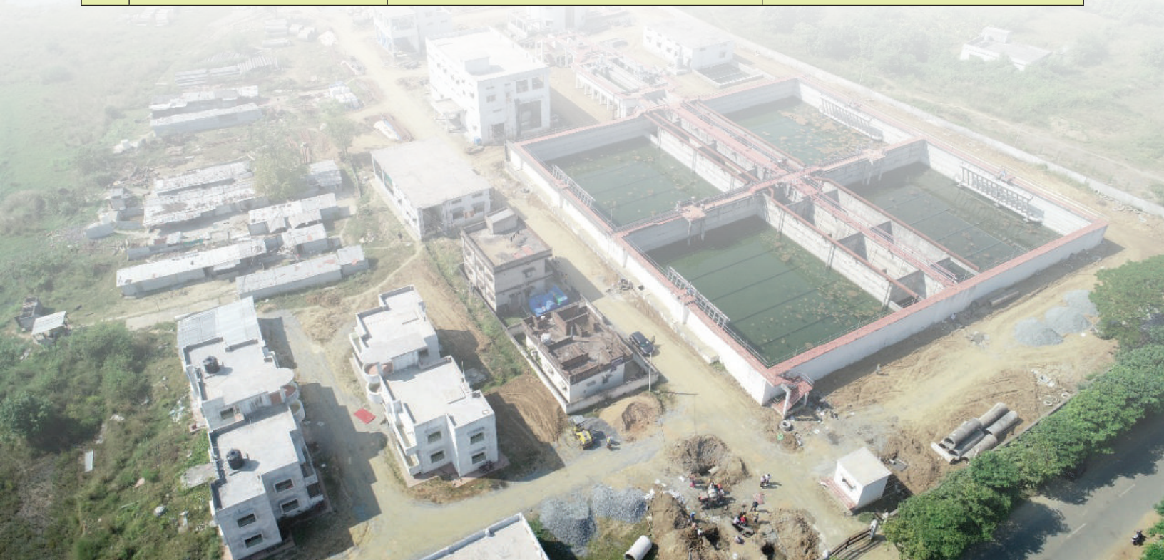
Sewerage Treatment Plant, Sambalpur
