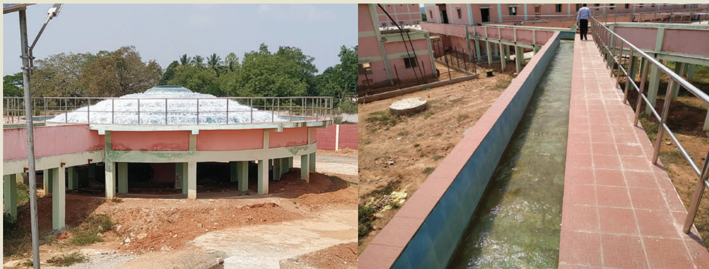
Bulk Water Supply Projects
