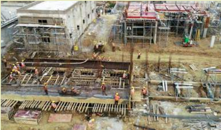
Construction of Primary Treatment Unit for Rourkela Sewerage Project
