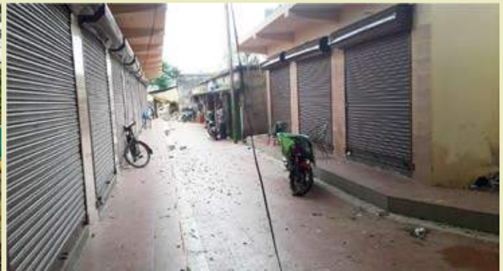
Construction of Meat Market at Unit-IV in Bhubaneswar
