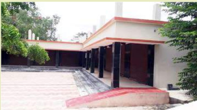
Construction of Meat Market at Ghatikia in Bhubaneswar
