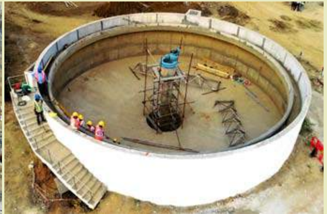
Construction of Gravity Sludge Thickener for Rourkela Sewerage Project
