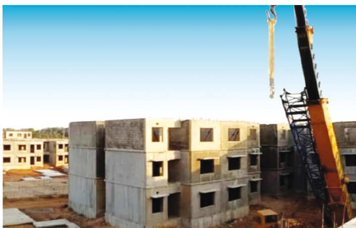
EWS Housing, Gadakana, Bhubaneswar
