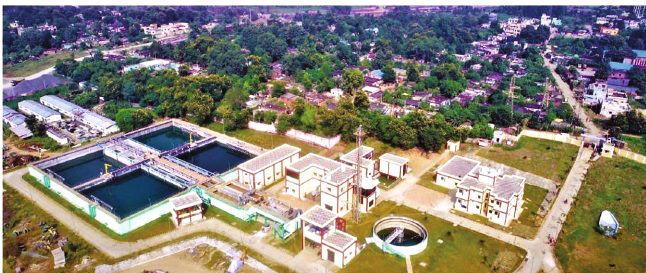
40 MLD Sewerage Treatment Plant, Rourkela
