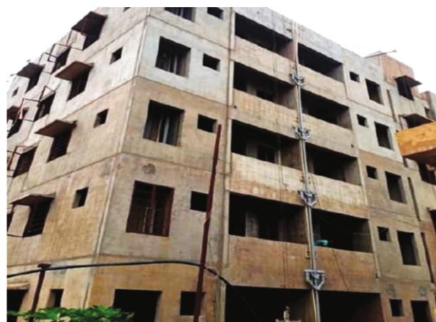
EWS Housing, Subudhipur, Bhubaneswar
